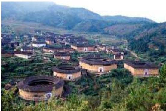
View of the Hakka Houses
